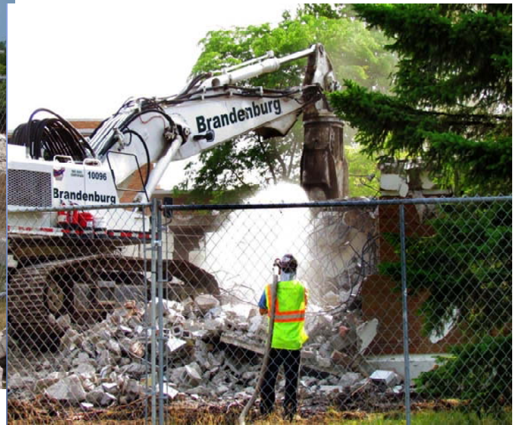
Restarting from the northwest corner to protect the big spruce. Spraying water to minimize dust.
