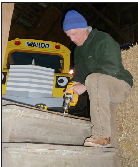
David Fawver, a regular volunteer at the EJC, installs a set of stairs for easy access to the Magic School Bus. The stairs were from the 1858 log cabin and were kept in storage in the granary when the cabin was taken down. Dennis Kornwolf who saved the stairs, must be smiling from above to see that they were put to good use!
