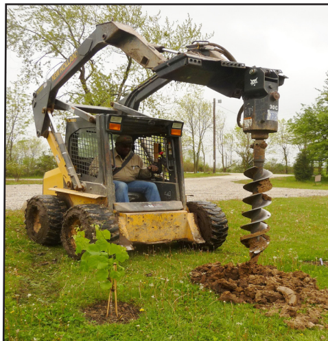
Eric Roberson and his nifty skidsteer makes easy work of digging the posts holes for the grape arbor project!
